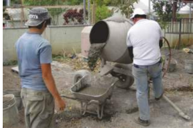
Figure preparing concrete with machine
